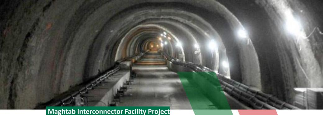
Laying of a single alternating-current cable by a Norwegian Company (Nexans) with a carrying capacity of 200 megawatts, linking Marina di Ragusa in Sicily to Magħtab. A new substation was built and linked to the Kappara distribution centre.
